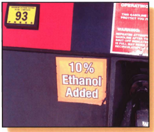
Figure 1.7. Ethanol, an alcohol derived from crops such as corn and sugar cane, is commonly added to gasoline, much like biodiesel is blended with regular diesel.
