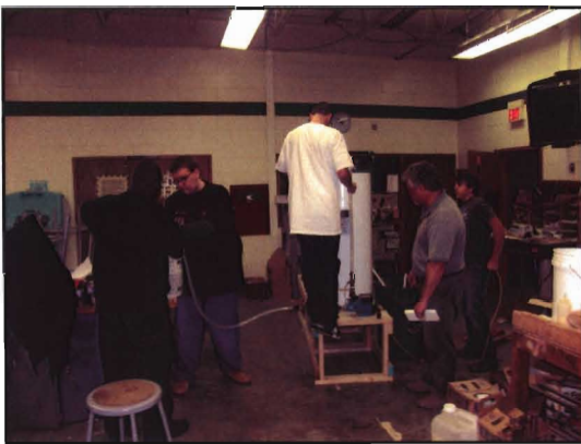
Figure 3.25. While Mr. Bullock looks on, students check the siphoning action of the pump by filling a pail of water and adjusting valves.
