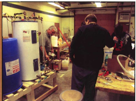
Figure 3.23. Mr. Bullock and students inspect the plumbing and installation of fluid pump, and then adjust pipe valves.
